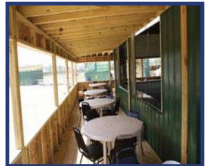
New Covered Pavillion Area
